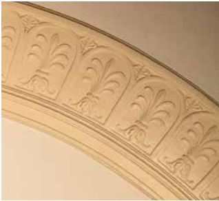
Ceiling, plaster, about 1910.
