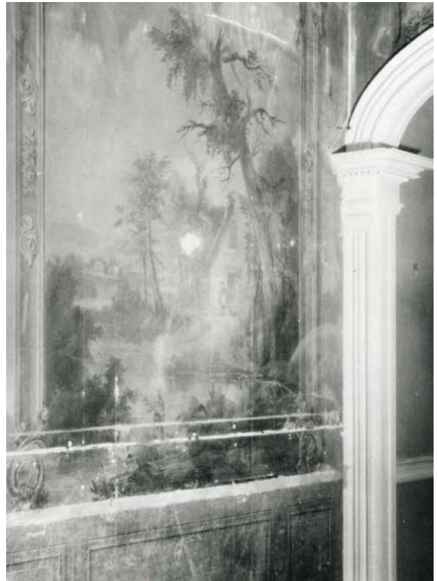
Mural, before restoration, 1931.
